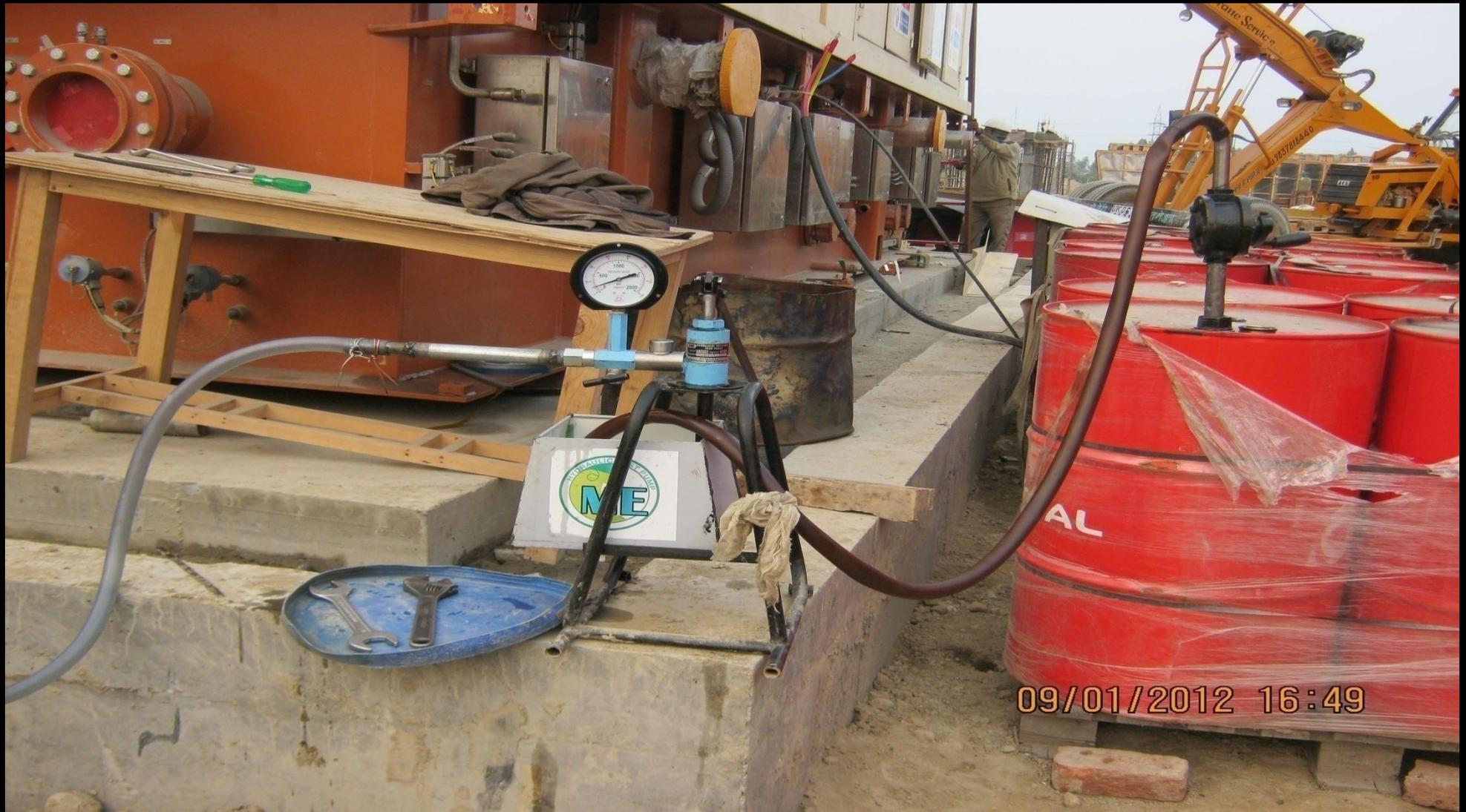
**MOT - oil filling before oil flushing**
